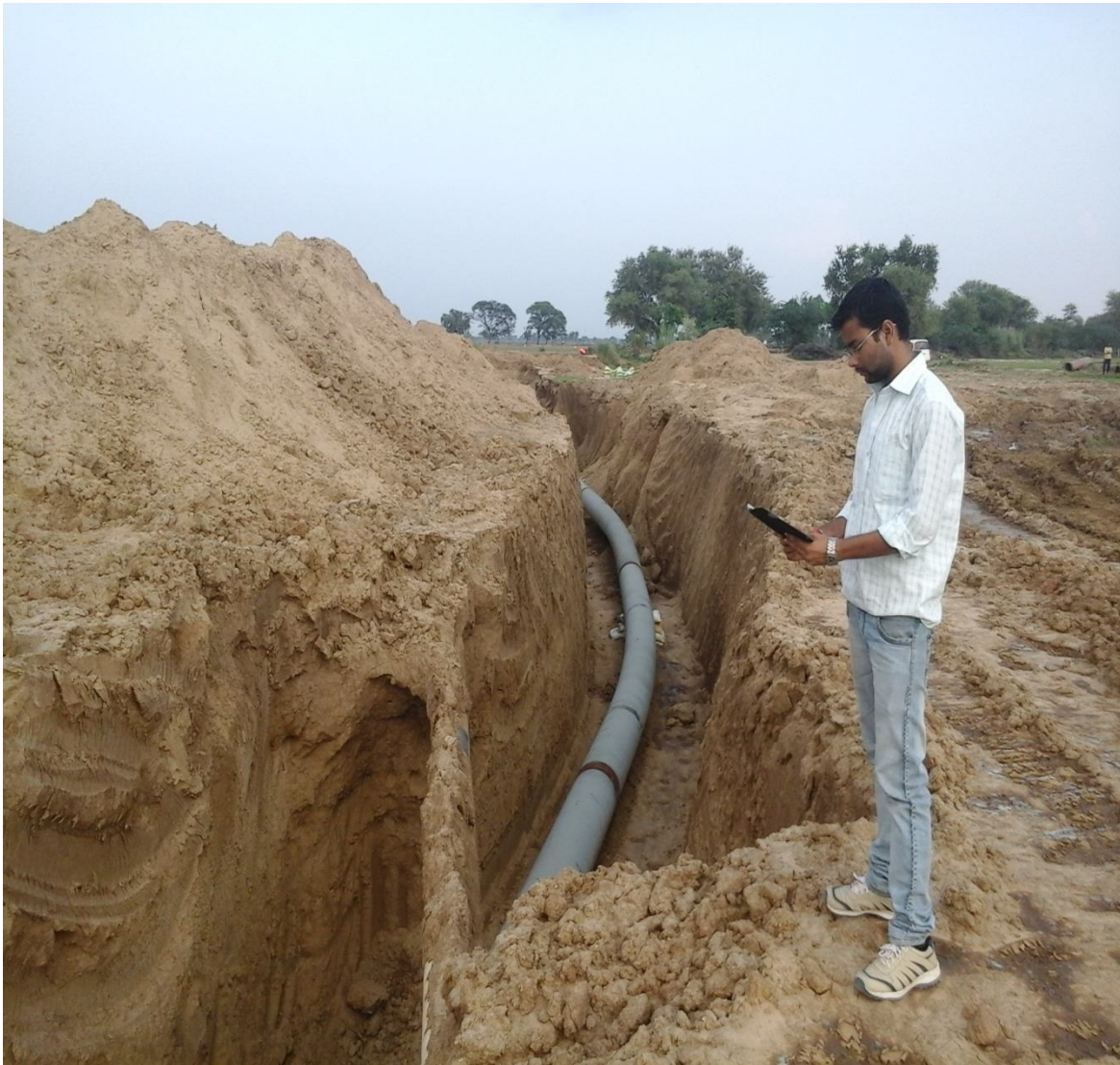
Site visit for borehole data collection
