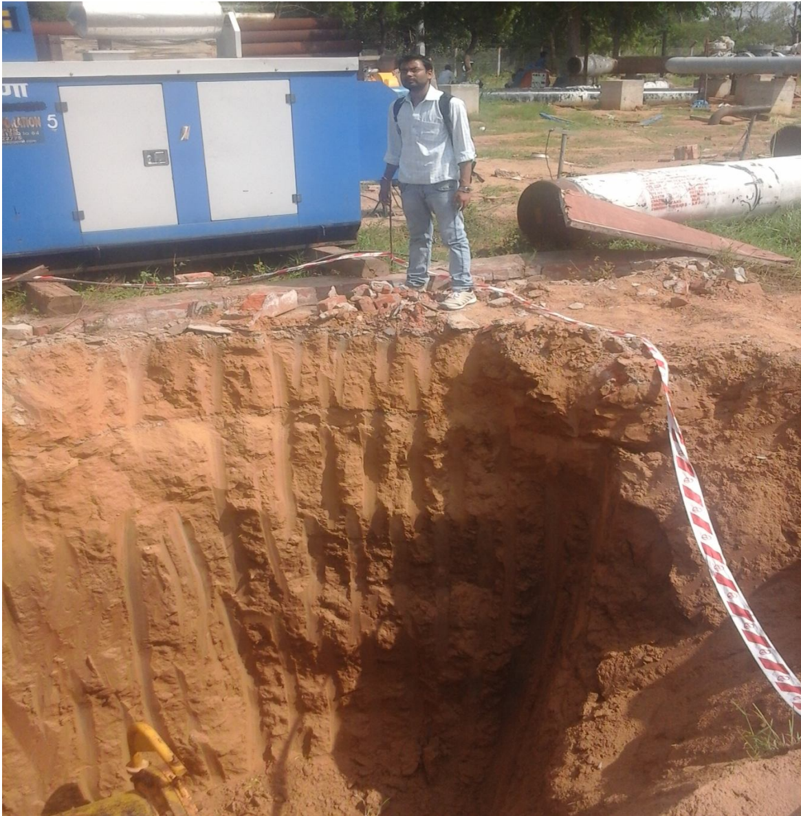
Excavation for laying pipes underground in delhi
